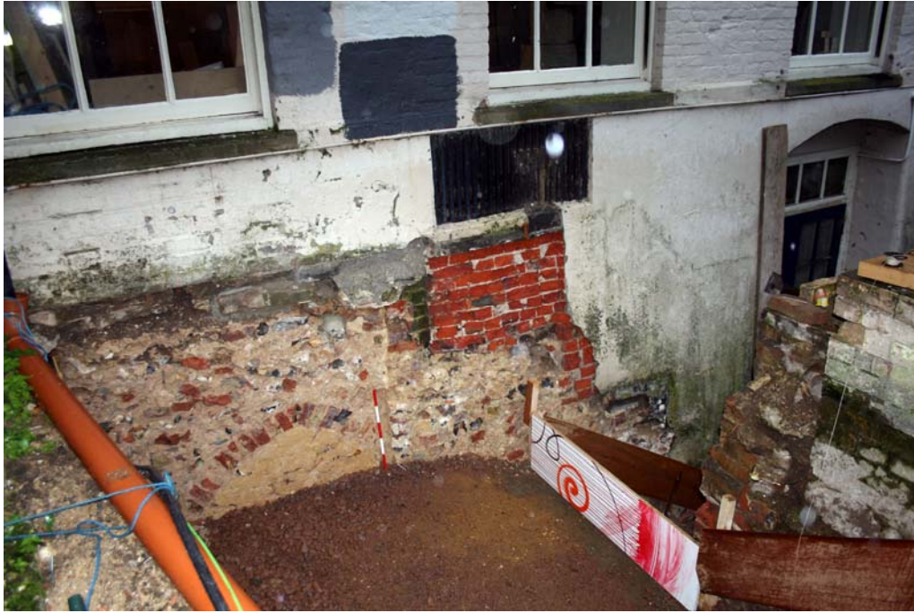
Plate 14. Blocked coal chute south of pointed arch facing south-west, 0.5m scale
