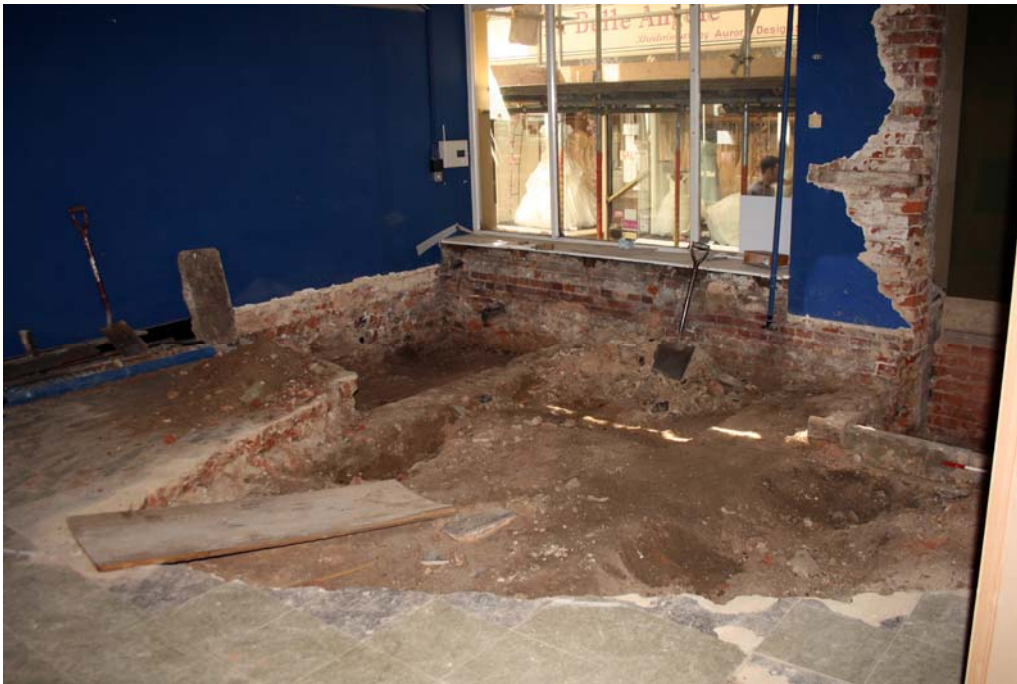
Plate 6. Foyer excavations facing south-west
