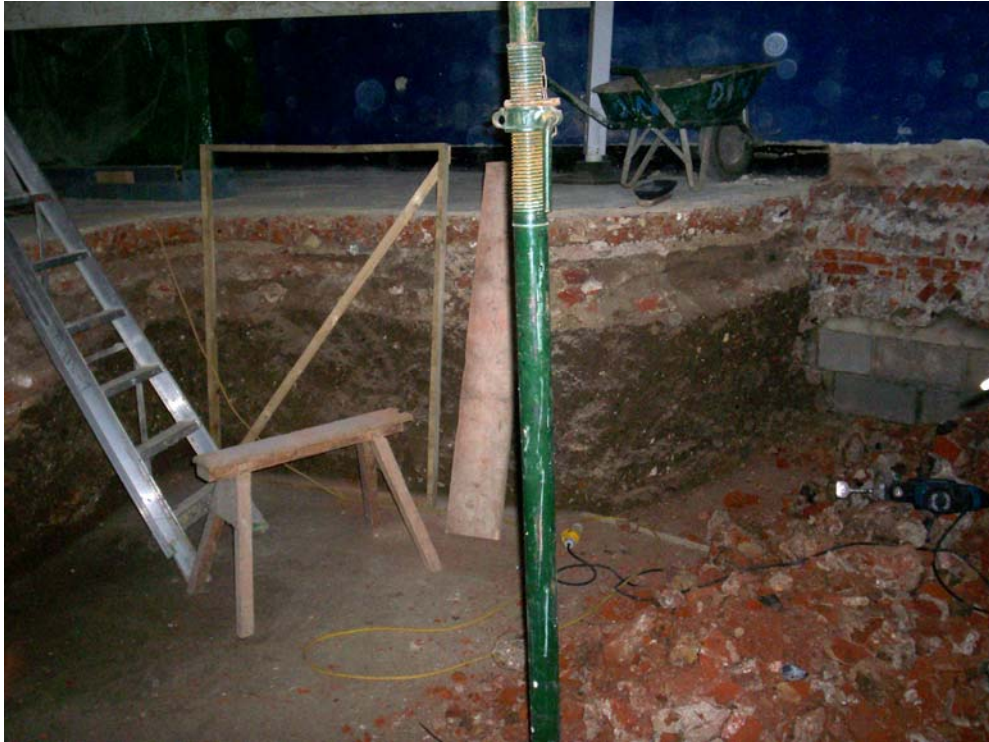
Plate 7. Foyer excavations west-facing section, facing south-east
