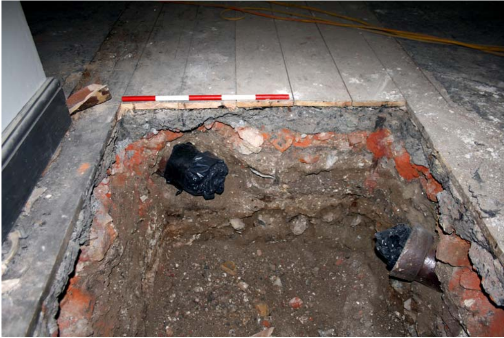
Plate 11. East-facing section of drainage junction, 0.5m scale
