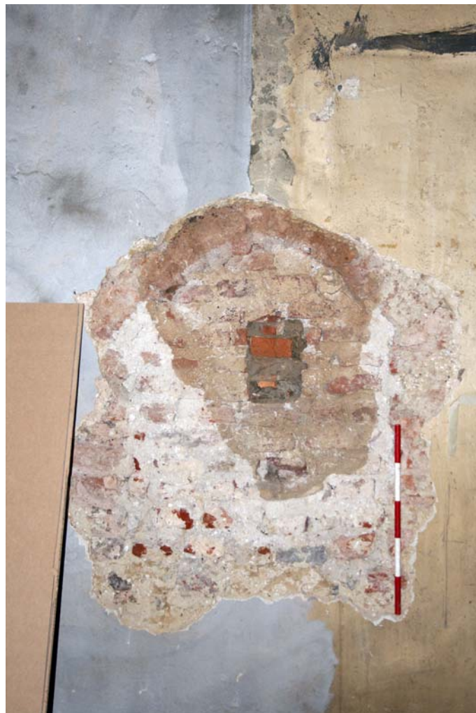
Plate 13. Four-centred arch revealed behind plaster on northern wall, 0.5m scale
