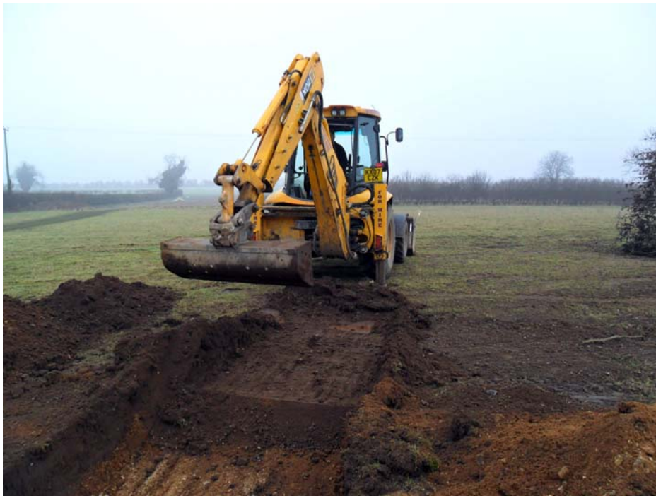
Plate 1. Machining the site, looking north
