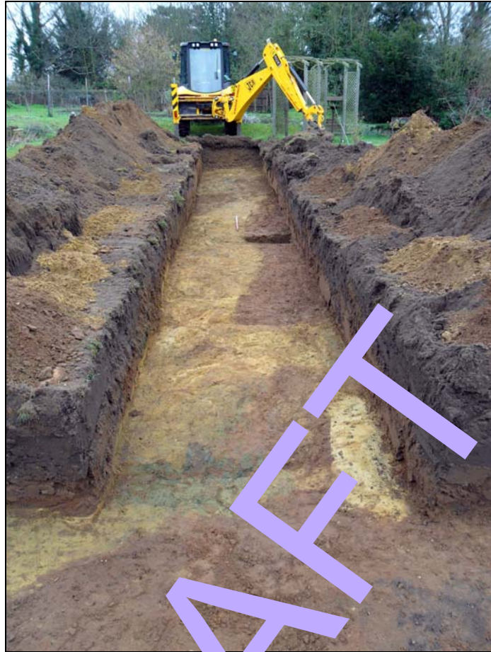
Plate 5. Trench 2, looking east
