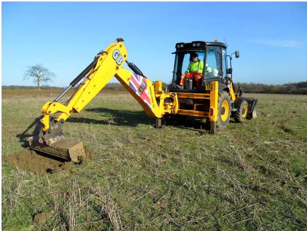
Plate 2. Machining, looking east
