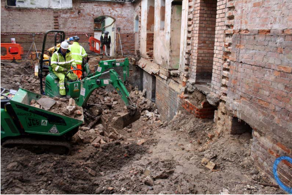
Plate 1. Removal of the under-floor heating system [9]
