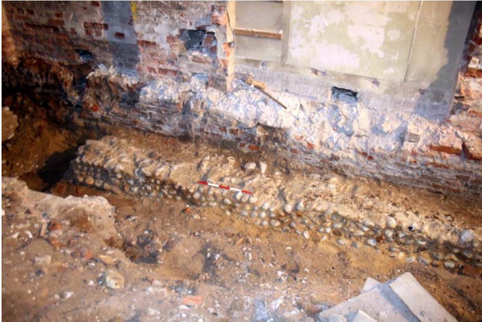
Plate 6. Wall [11] as observed in Room D (looking south-west)
