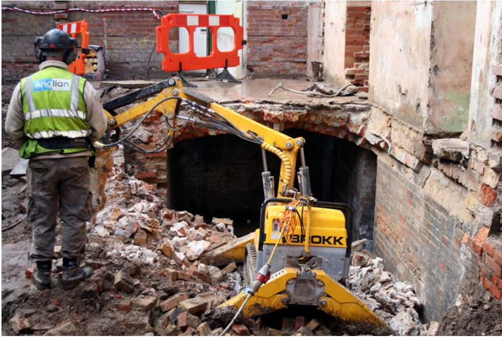
Plate 4. Cellar [12] being demolished
