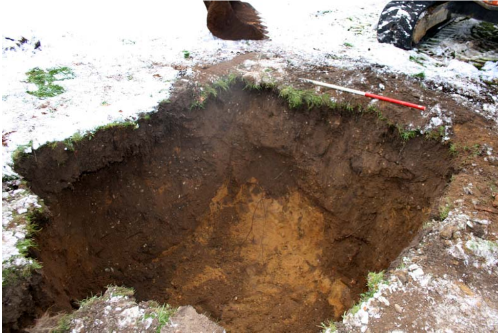
Plate 2. East-facing section of water tank pit, 1m scale
