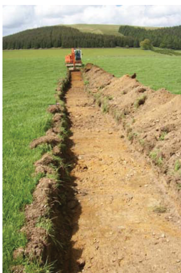
Plate 1: Trench 7 from SE
