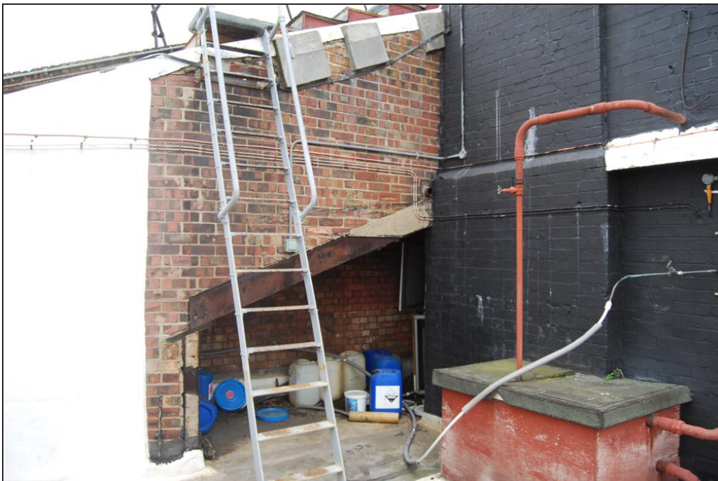
Plate 33: Roof at Rear
