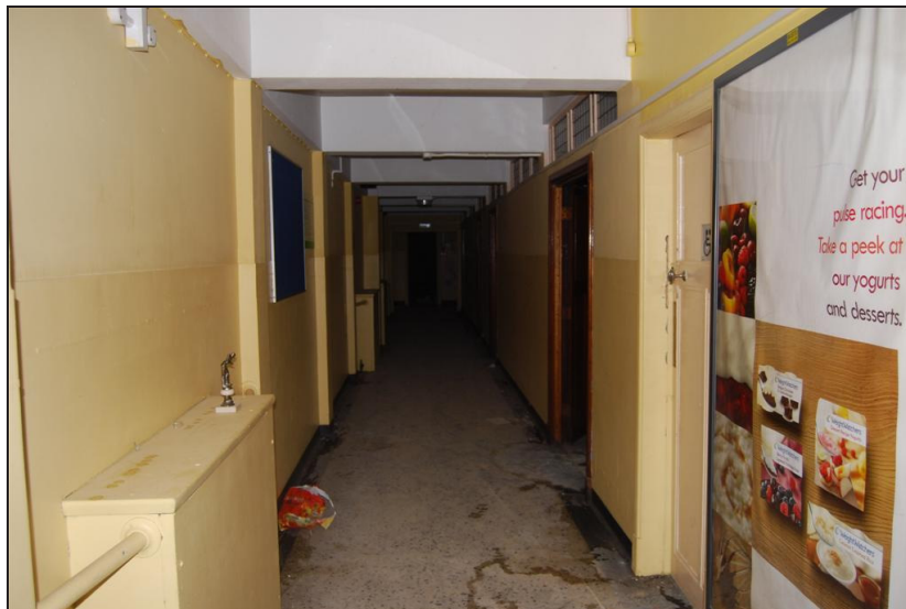
Plate 48: Room G17 Looking West
