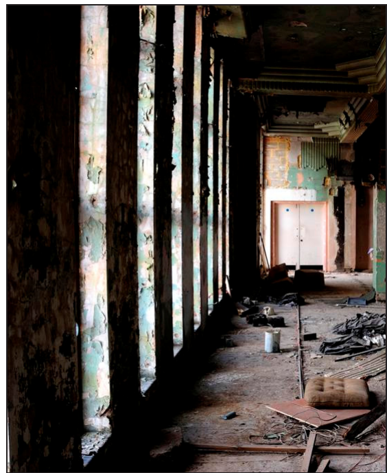
Plate 24: View of Function Room Looking South
