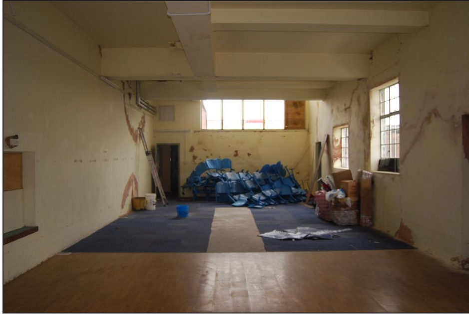
Plate 32: View South of Second Floor of Ice Rink, Rear Block
