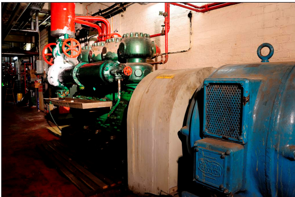
Plate 29: Second Compressor Manufactured by L. Sterne and Co Ltd, Crompton Parkinson Motor in foreground.
