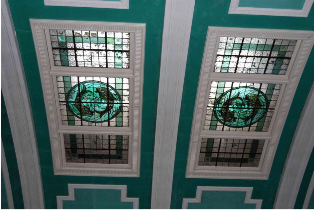
Plate 42: Pair of Glazed Roof Panels
