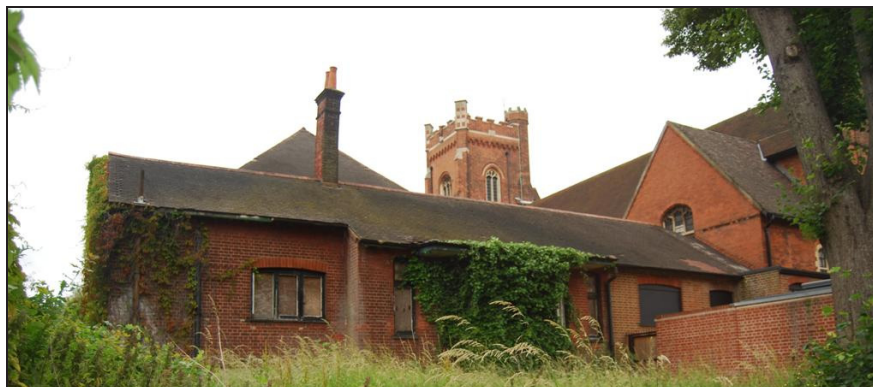
Plate 10: Ancillary Block, View Looking Southeast
