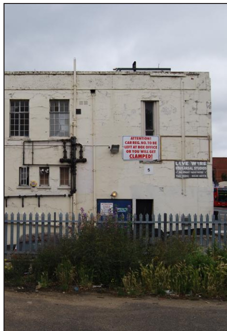
Plate 20: External View Including Stairwell Window
