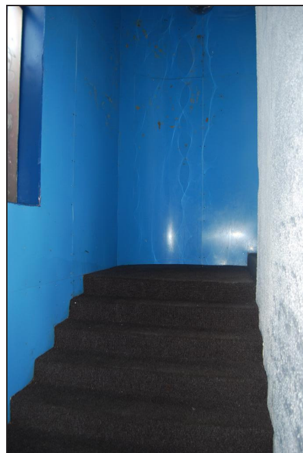
Plate 21: Corner Stairwell Leading To First Floor
