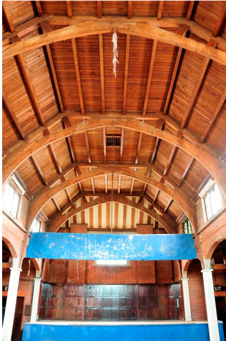
Plate 9: View of Roof Assemblies
