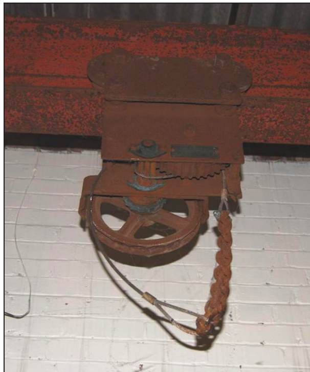
Plate 30: Hoist over basement trap doors.
