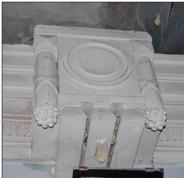
Plate 45: Corbel Detail, Roof Assembly.
