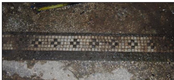
Plate 3: Lobby Floor Detail
