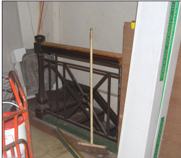
Plate 54: Stair Railing to Rear
