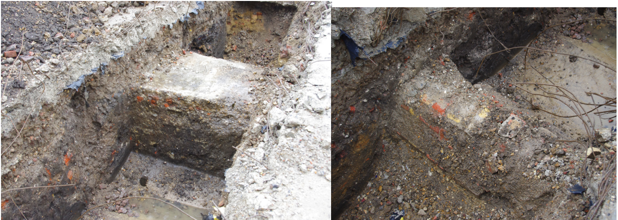
Plate 1 – Concrete base [104] and wall [105]
