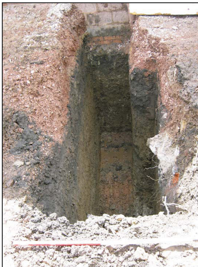
Trench 2 - looking south
