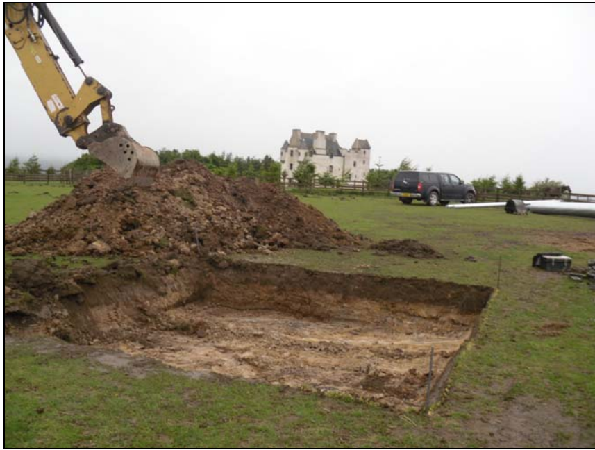
Plate 1: View of excavation of turbine foundation base
