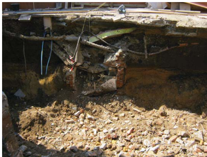
Plate 4 – Western exposed section showing (4), (3) and structure [2].
