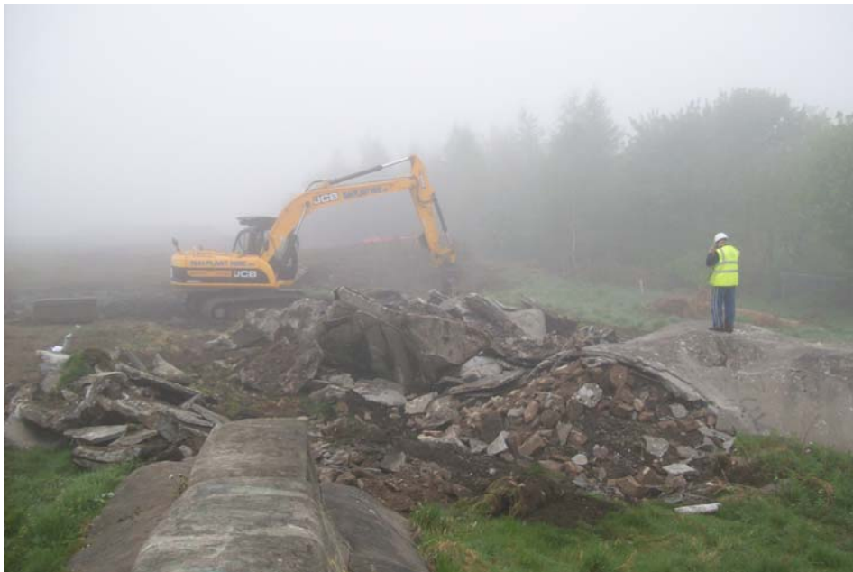
Plate 10: Gulliver during demolition
