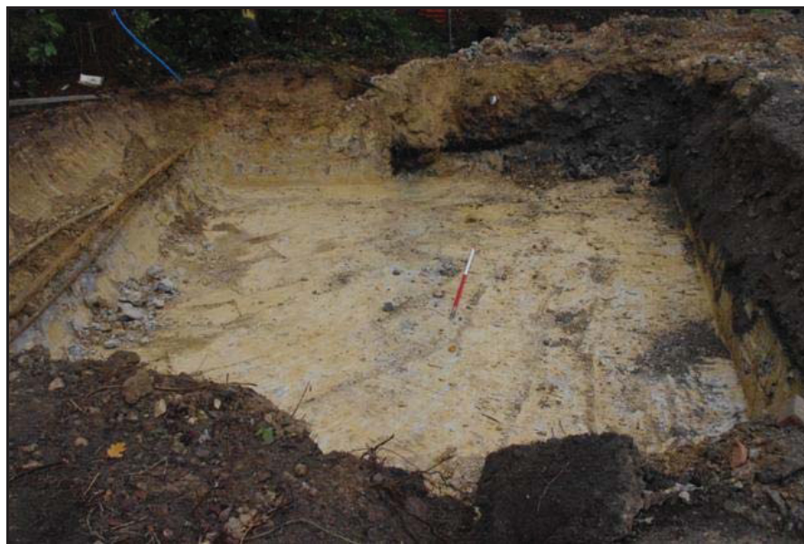
Plate 2: Trench 1 - sub-station excavations (direction south)
