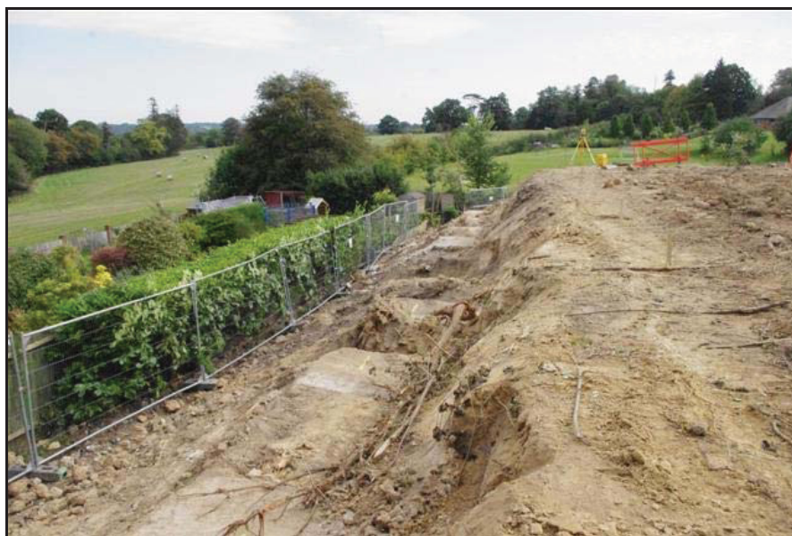
Plate 1: Northern limit of site – illustrating made-ground deposits (direction north-east)
