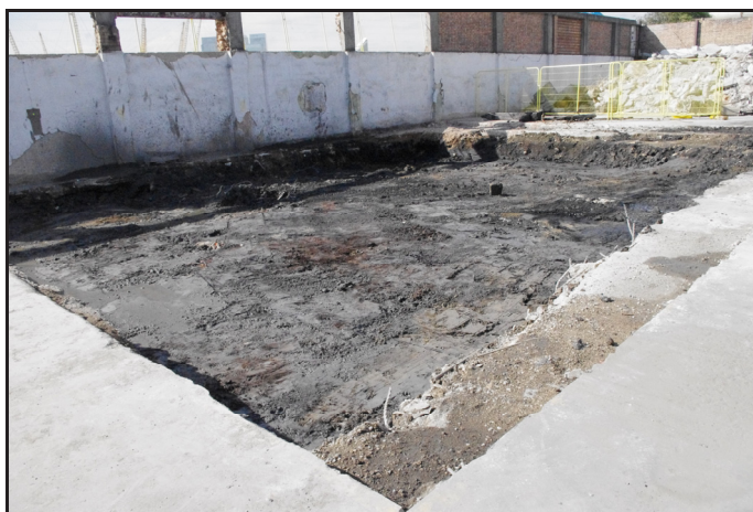
Plate 3. Post excavation view of watching brief area, looking north-west
