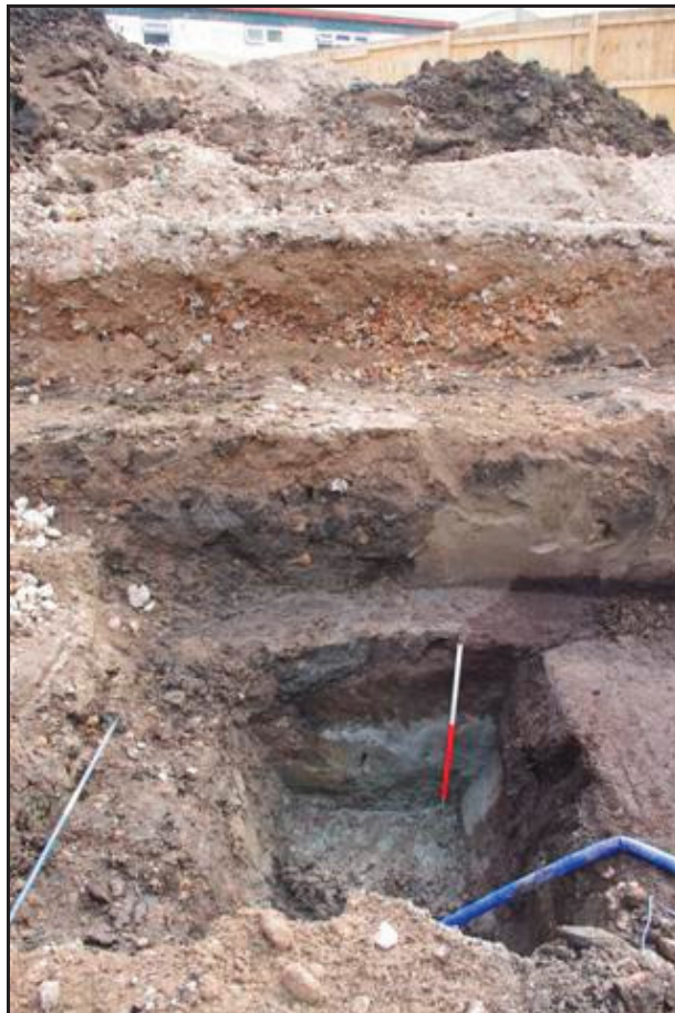
Plate 3: Trench 1 – Section 1 full sequence from natural sands (105) to modern Made Ground (100), direction south-east
