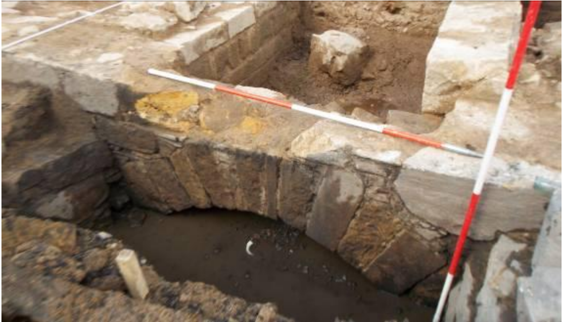
Plate 3; external view of arch (1052) from the south-east
