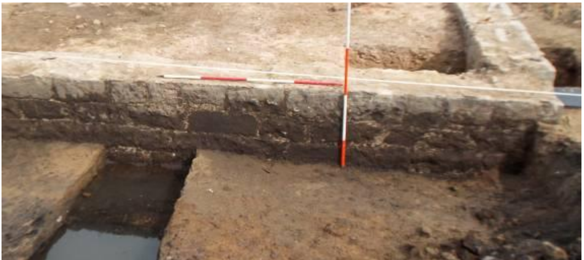
Plate 2; Wall (1053) from the west
