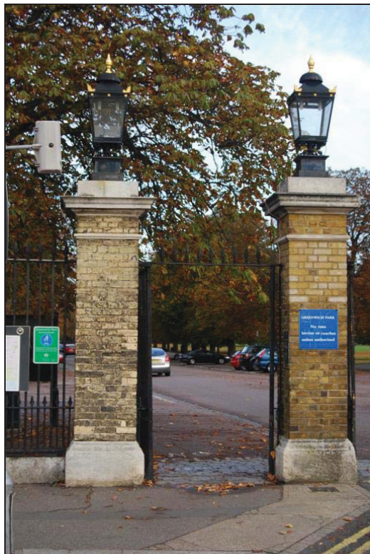
Plate 4: West Pair of Piers
