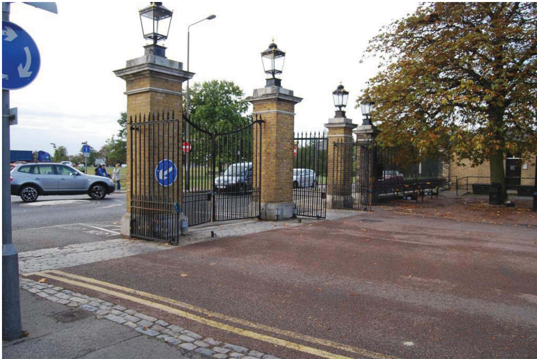
Plate 6: Oblique View of Blackheath Gates
