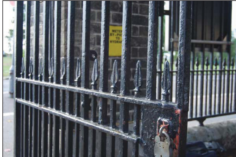
Plate 9: Spear Point Detail of Gate Lock Rail
