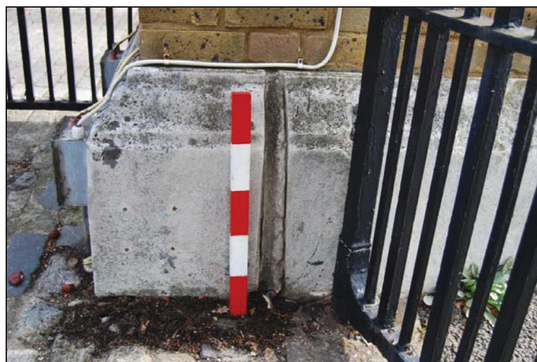
Plate 2. Incised Route for Previous Cabling
