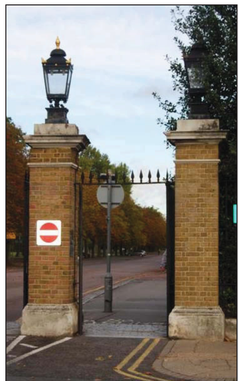
Plate 5: East Pair of Piers
