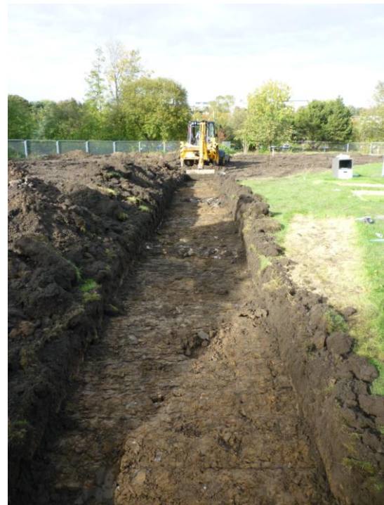
Plate 4: Trench 4 from south
