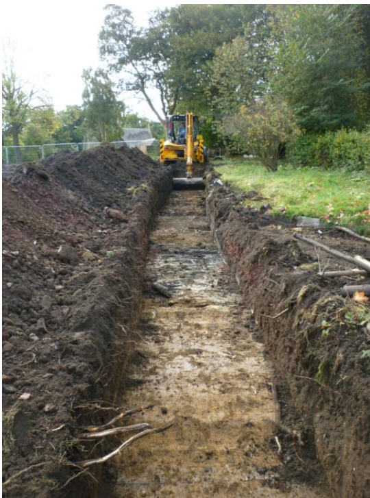
Plate 3: Trench 2 from north
