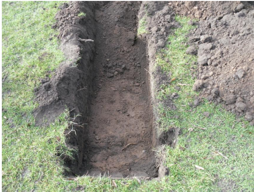
Plate 1: Working shot of a site investigation pit under excavation
