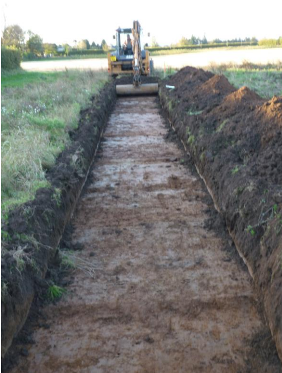
Plate 1: Trench 1 from north
