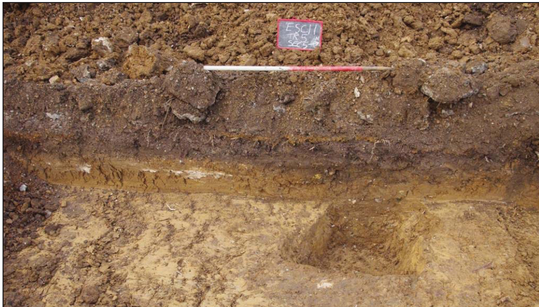
Plate 3: Trench 5, Looking West
