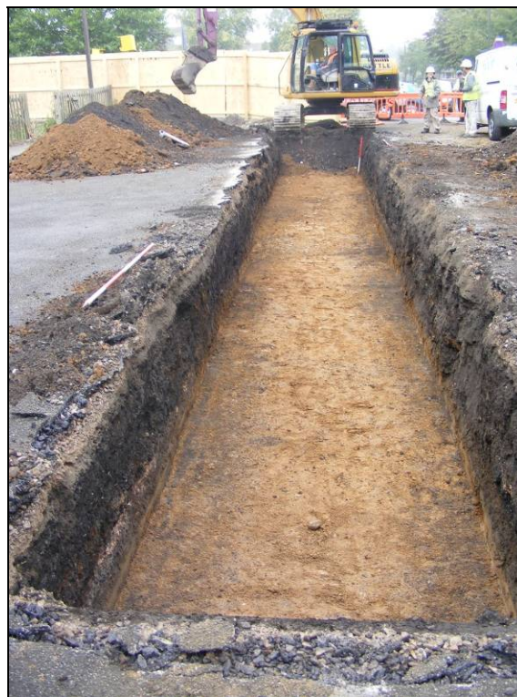
Plate 4: Trench 3 looking north west.
