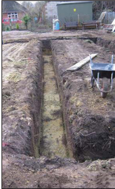
Plate 2: Excavated foundation trench (direction west)
