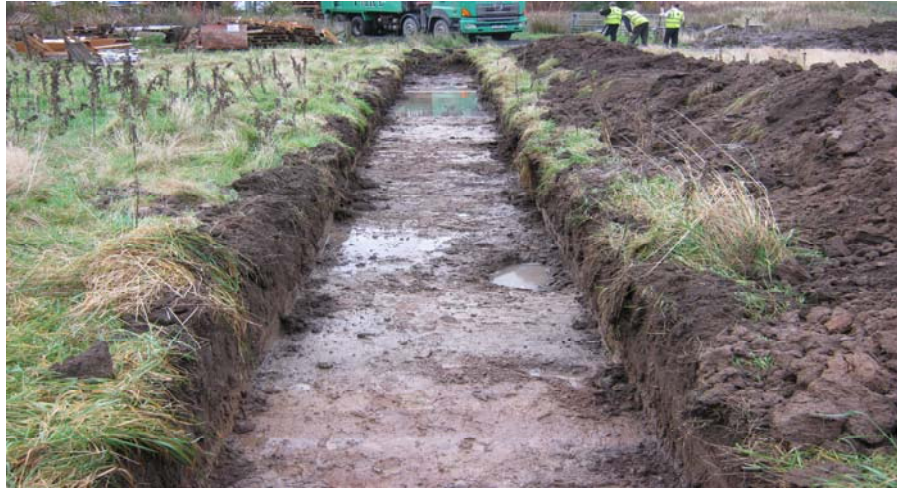
Plate 1: Trench 1 Post-excavation from East
