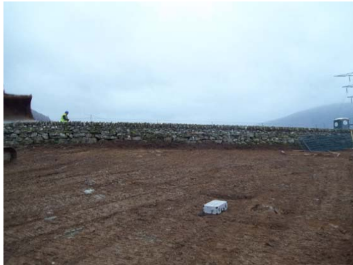
Plate 1: W Elevation of Wall 22 (i)
