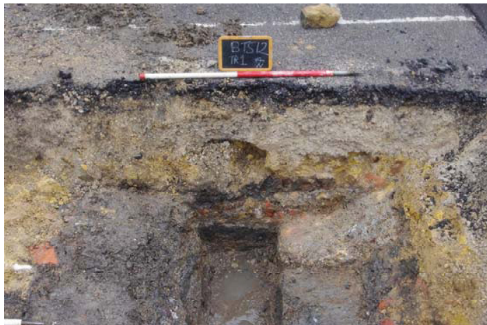
Plate 1 – Made ground deposits and concrete base (104).
