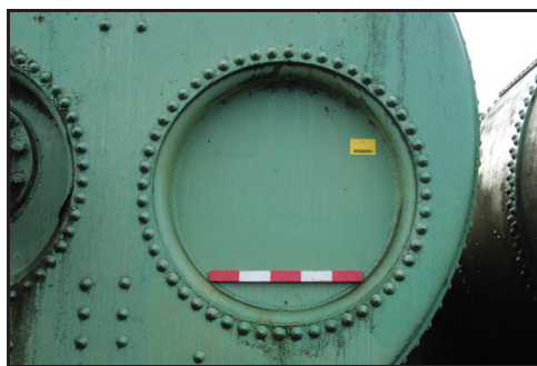
Plate E. Detail of Sealed Opening Tank 5 Northwest Elevation Looking Southeast
