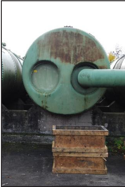
Plate J. Tank 2 Northwest Elevation Looking Southeast
