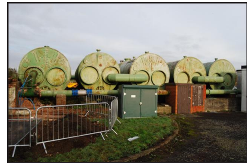
Plate D. Southeast Elevation of Tanks Looking North
