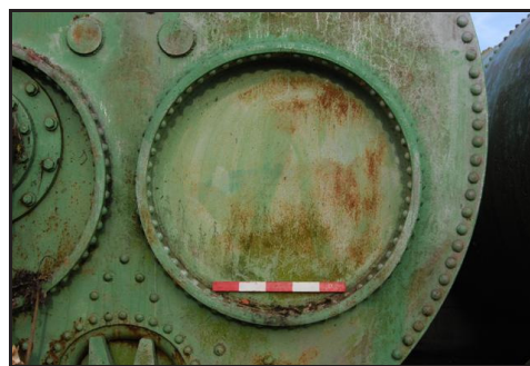
Plate F. Detail of Sealed Opening Tank 1 Southeast Elevation Looking Northwest
