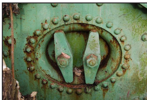
Plate G. Detail of Bolted Attachments Tank 1 Southeast Elevation Looking Northwest
