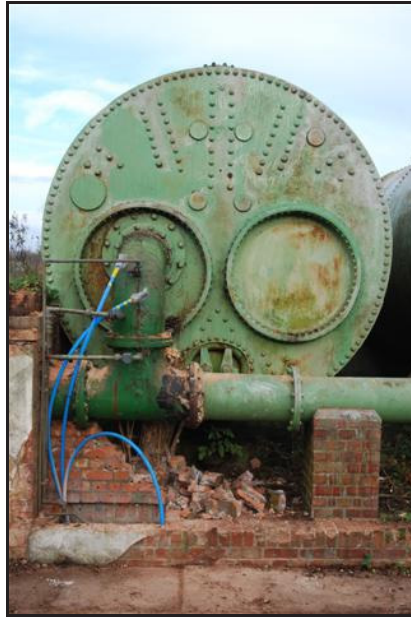
Plate H. Tank 1 Southeast Elevation Looking Northwest
