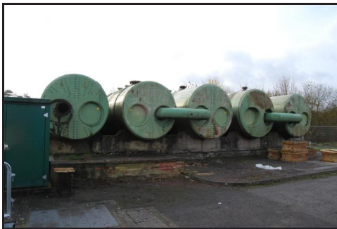
Plate C. Northwest Elevation of Tanks Looking South
