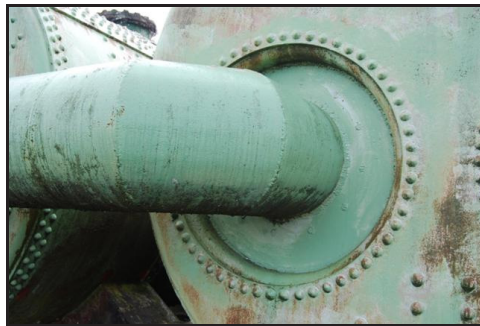
Plate I. Tank 3 Detail of Sealed Opening Northwest Elevation Looking East
