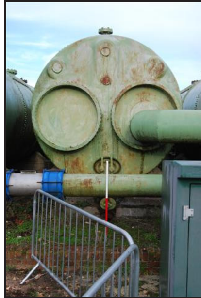
Plate K. Tank 2 Southeast Elevation Looking Northwest
