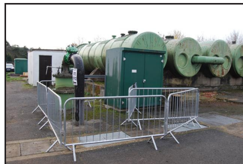
Plate P. Northern Kiosk Looking South
