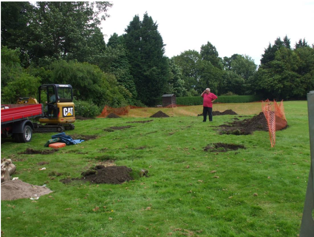
Plate 1 – Foundation pad excavations for temporary building from south
