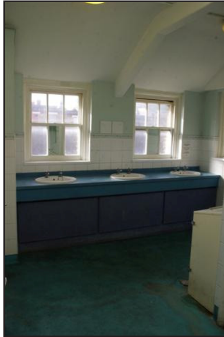
Plate 27: Room S23 Looking South
