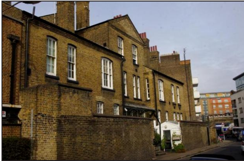
Plate 3: St. Mungo's Building Looking North
