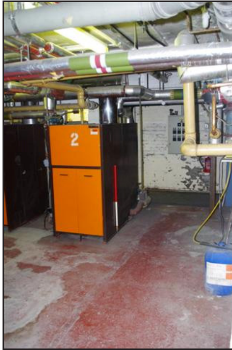
Plate 20: Room B13 Looking West
