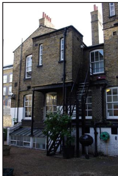
Plate 6: First Floor Extension Looking East
