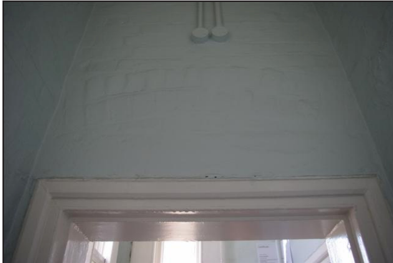
Plate 26: Detail of Window Arch Room F5 Looking Southeast
