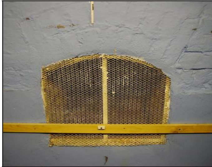
Plate 22: Detail of Coal Hole Room B15 Looking Southeast
