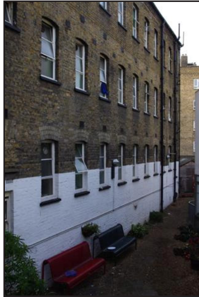
Plate 4: Northeast Elevation Looking West
