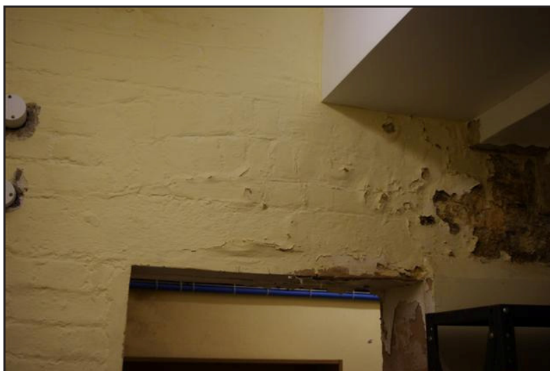
Plate 21: Partially Blocked Arch Room B2 Looking North
