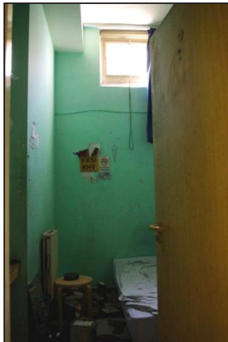
Plate 11: Room G23 Looking Northeast
