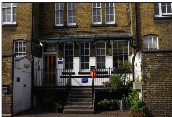
Plate 15: Detail of Southeast Elevation Looking Northwest
