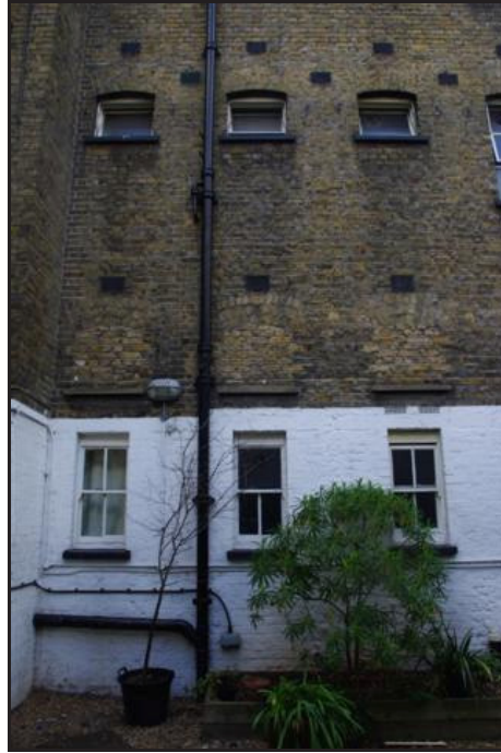
Plate 7: Blocked Windows to Northeast Elevation Looking Southwest
