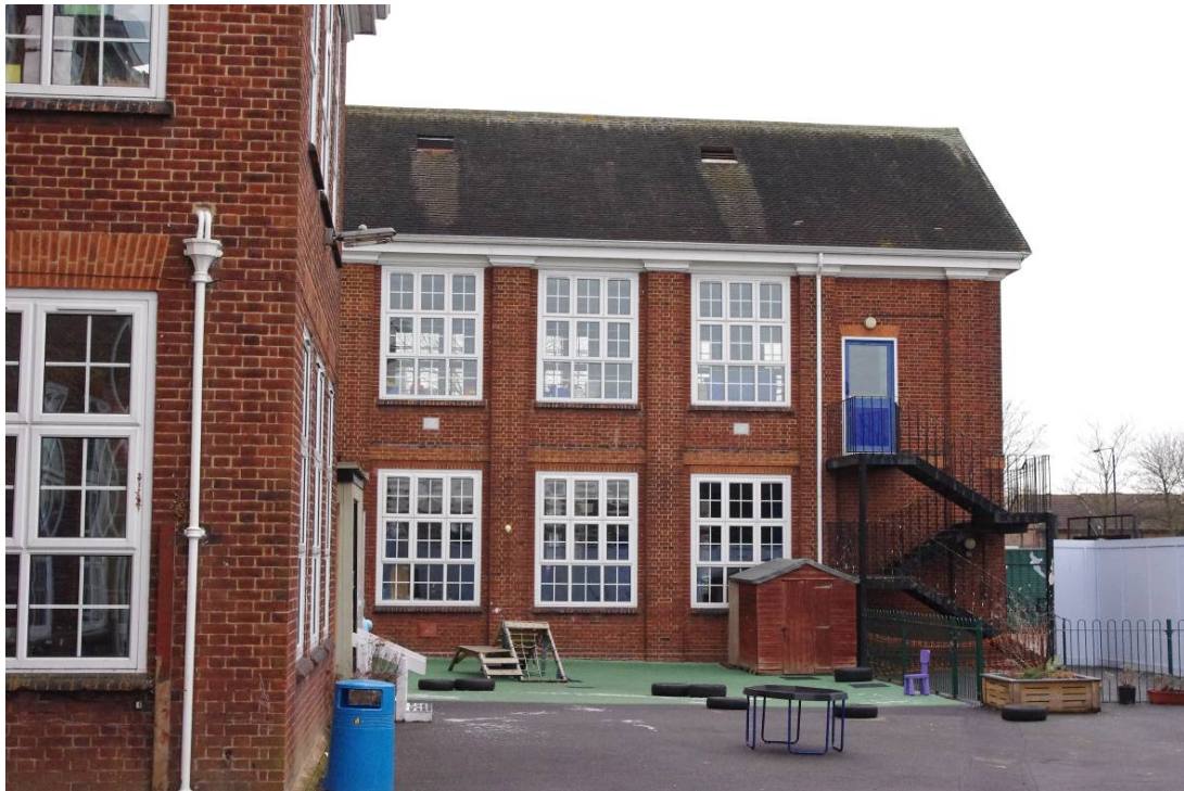
Plate 5. Area of extension to rear of original school block (Block 1), looking west.
