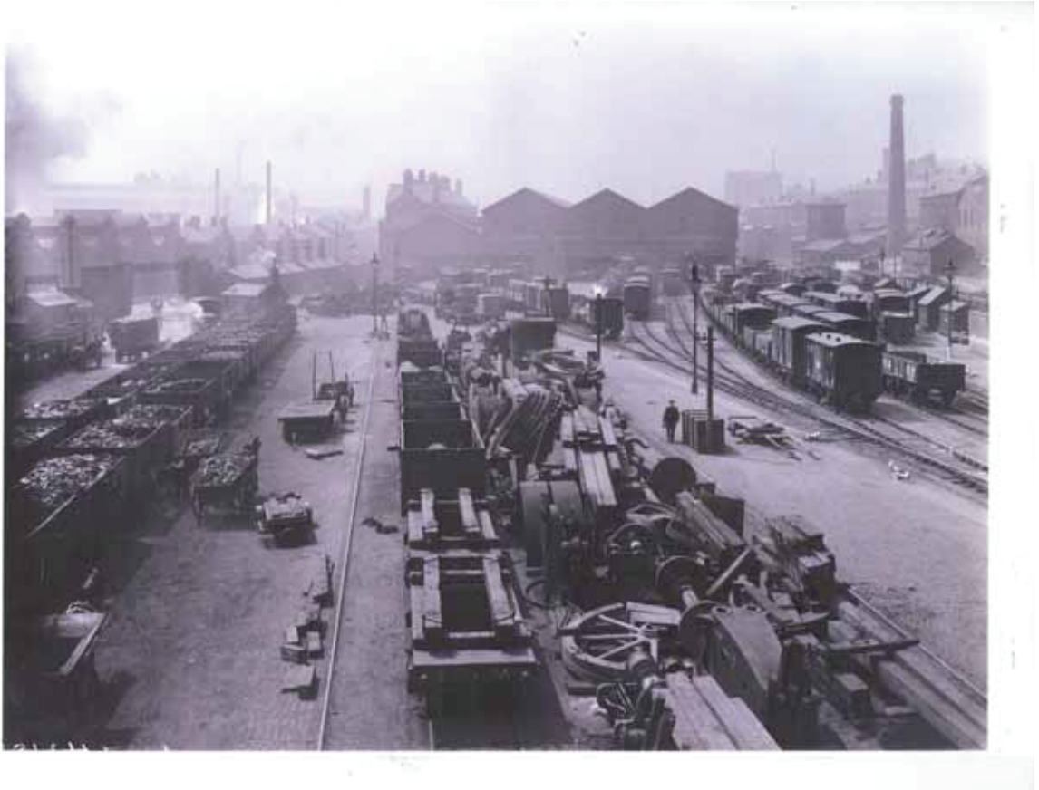
Plate 6: View of Midland Railway Goods Yard 1912, showing the Electric Light Station building on the far right
