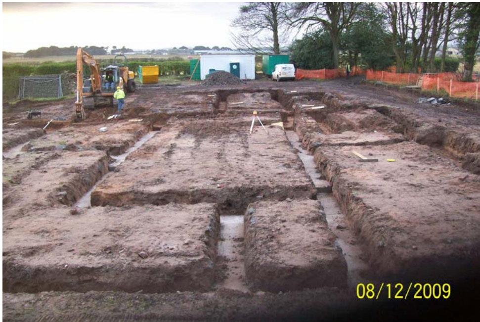
Plate 2 View of foundations of new build during from East
