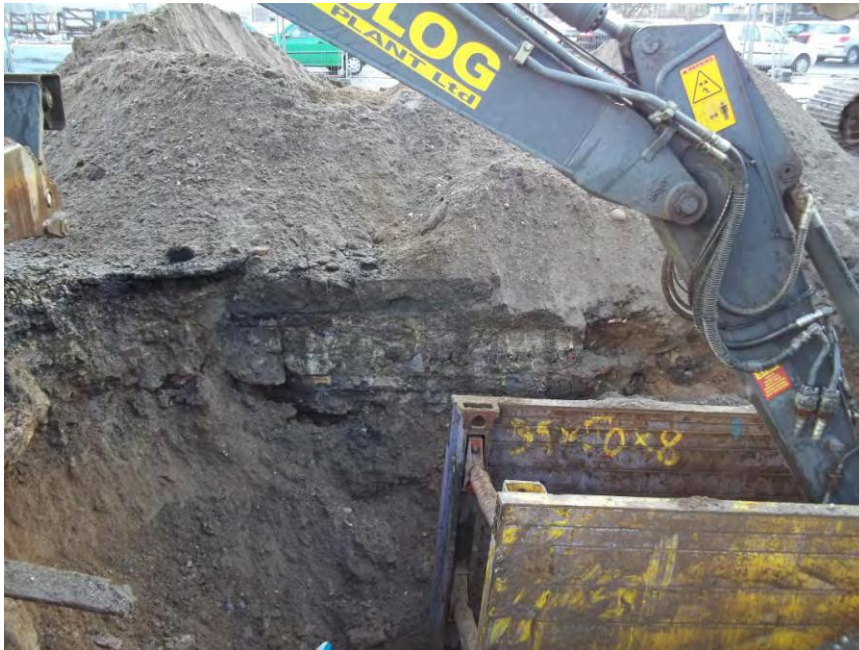
Plate 3 - An example of modern foundations throughout the site
