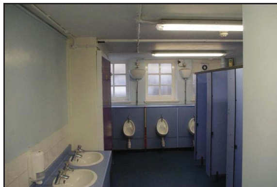
Plate 9: Room 4 Looking South
