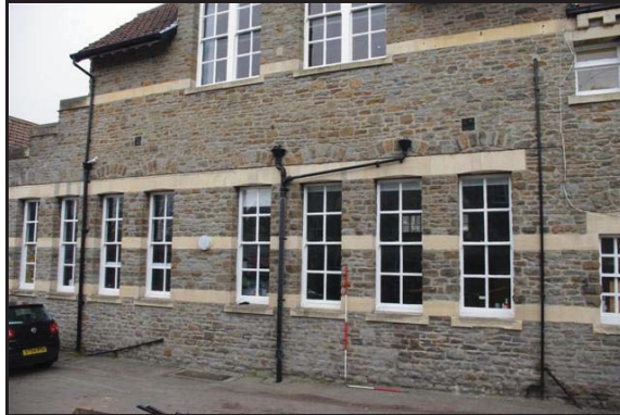
Plate 3: Western Elevation of Building B Looking Northeast
