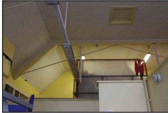
Plate 18: Room 16 Looking North
