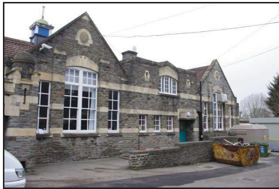
Plate 2: Eastern Elevation of Building A Looking Northwest
