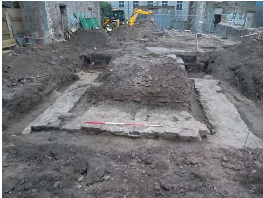
Plate 2: Vestry Foundations [001] and Wall [002].
