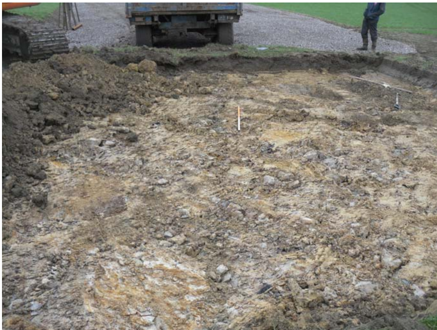
Plate 1 - Post excavation shot of turbine base showing rubble drain
