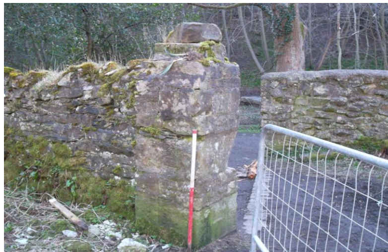
Plate 9: Wall 1 Main Entrance from North
