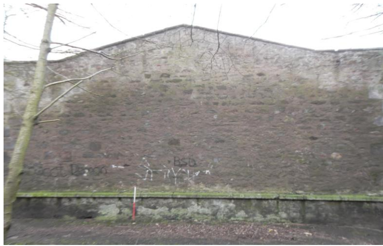
Plate 4: Doocot Rear Elevation from North
