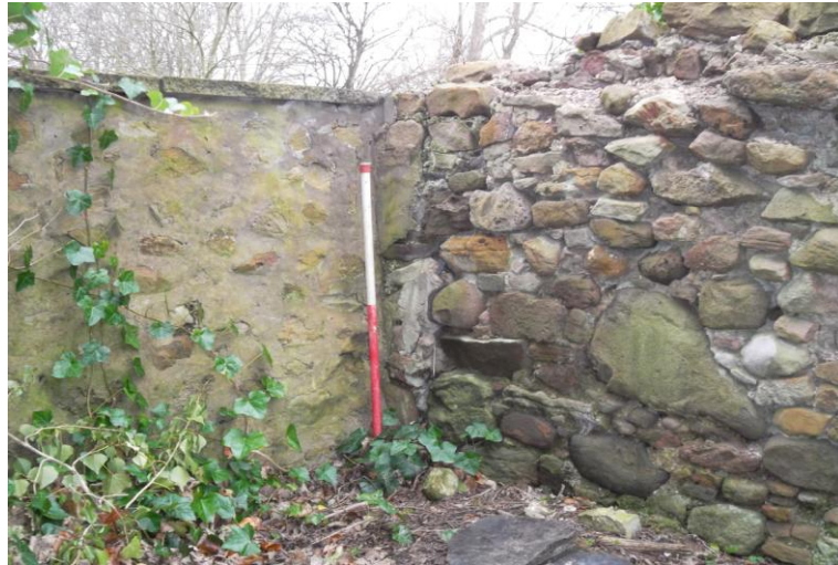
Plate 6: Wall 1 north-east corner from South-west
