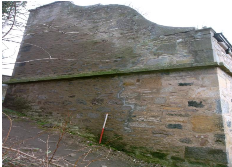
Plate 3: Doocot Western Elevation from South-west
