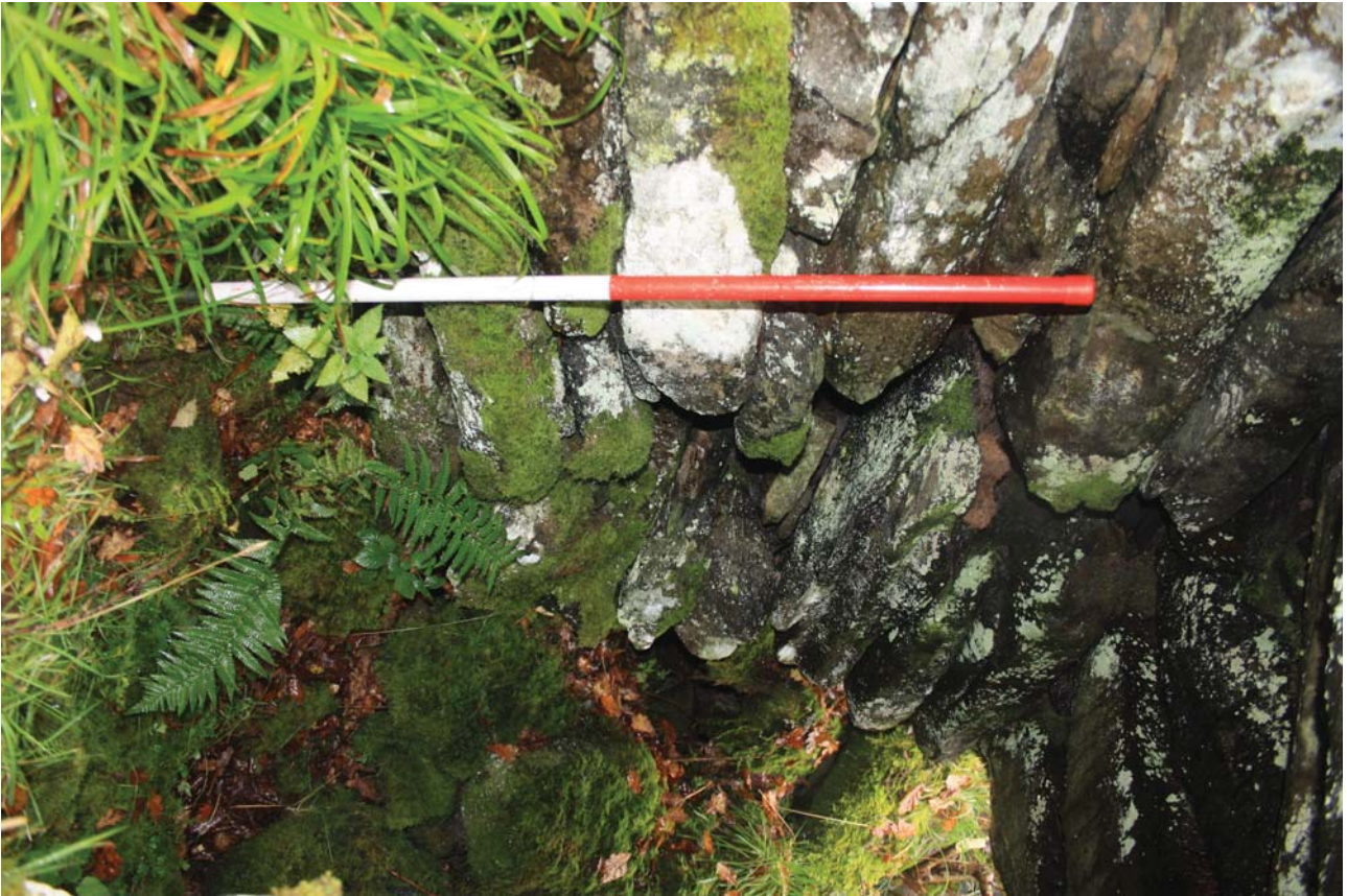
Plate 13: View of the stonework in the entrance to the guard cell, facing E
