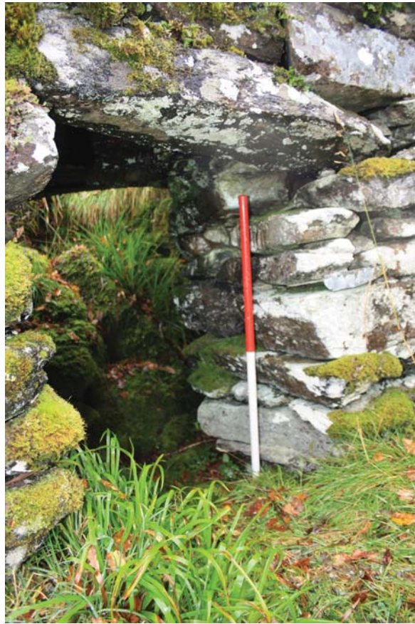
Plate 9: Entrance to guard cell in NW-facing elevation of S entrance
