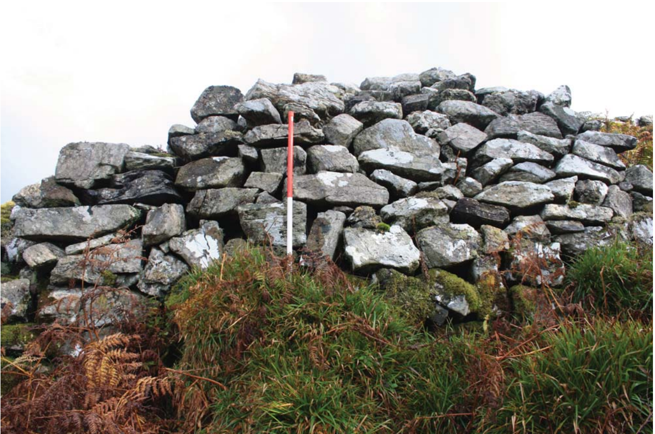
Plate 41: Outer wall face of dun 3, at point 10, facing E
