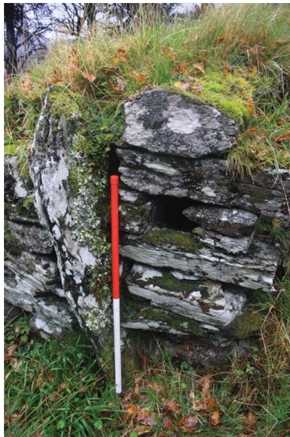
Plate 6: Bar hole in SE-facing elevation of entrance, behind door jamb
