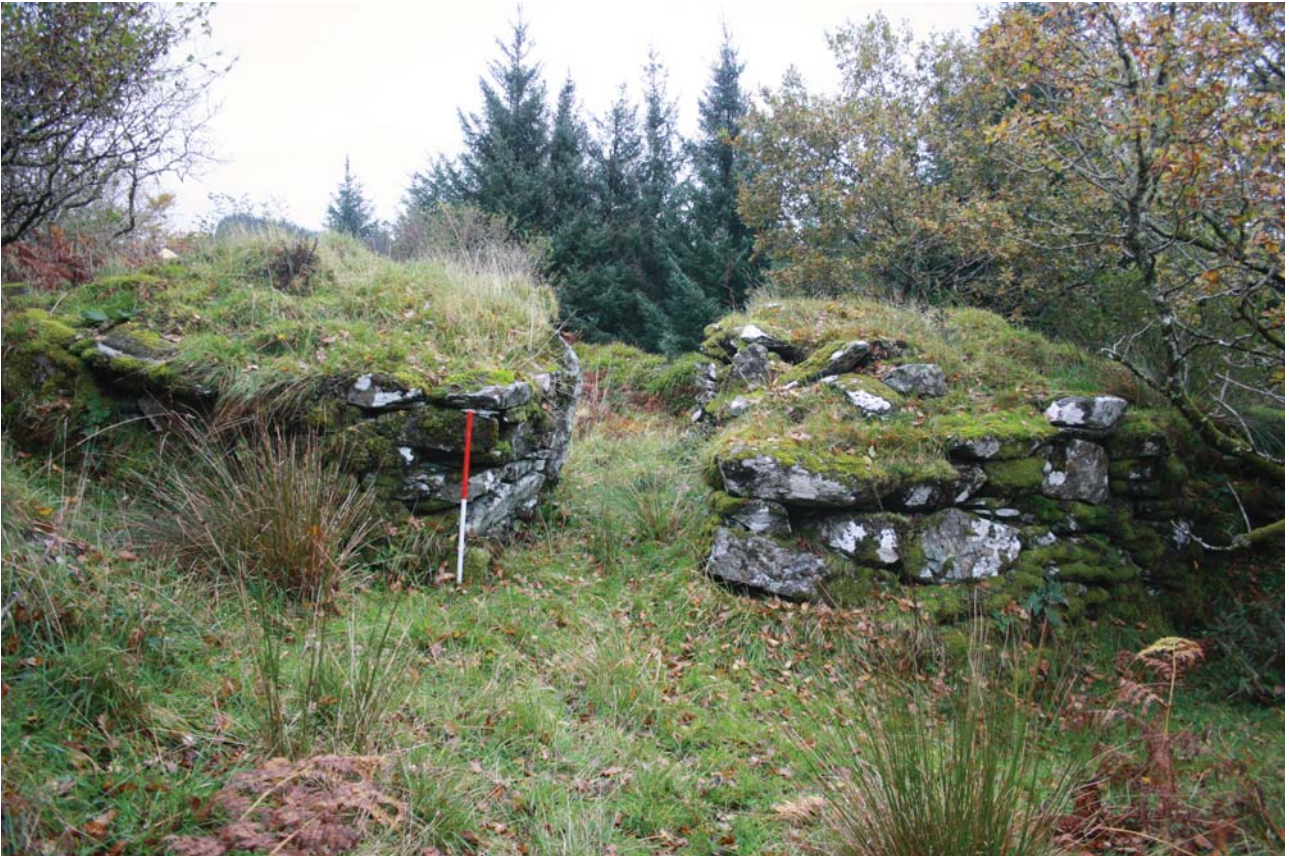
Plate 1: General view of the S entrance to Druim an Duin, facing north
