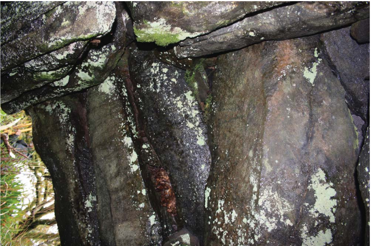
Plate 14: View of the lintels capping the guard cell in the southern entrance
