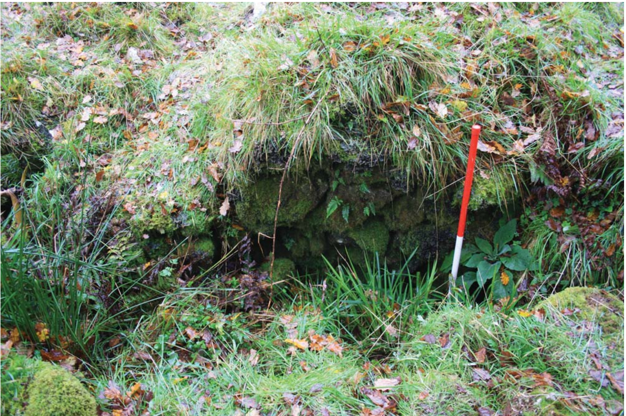
Plate 12: Exposed stonework in the guard cell, facing N
