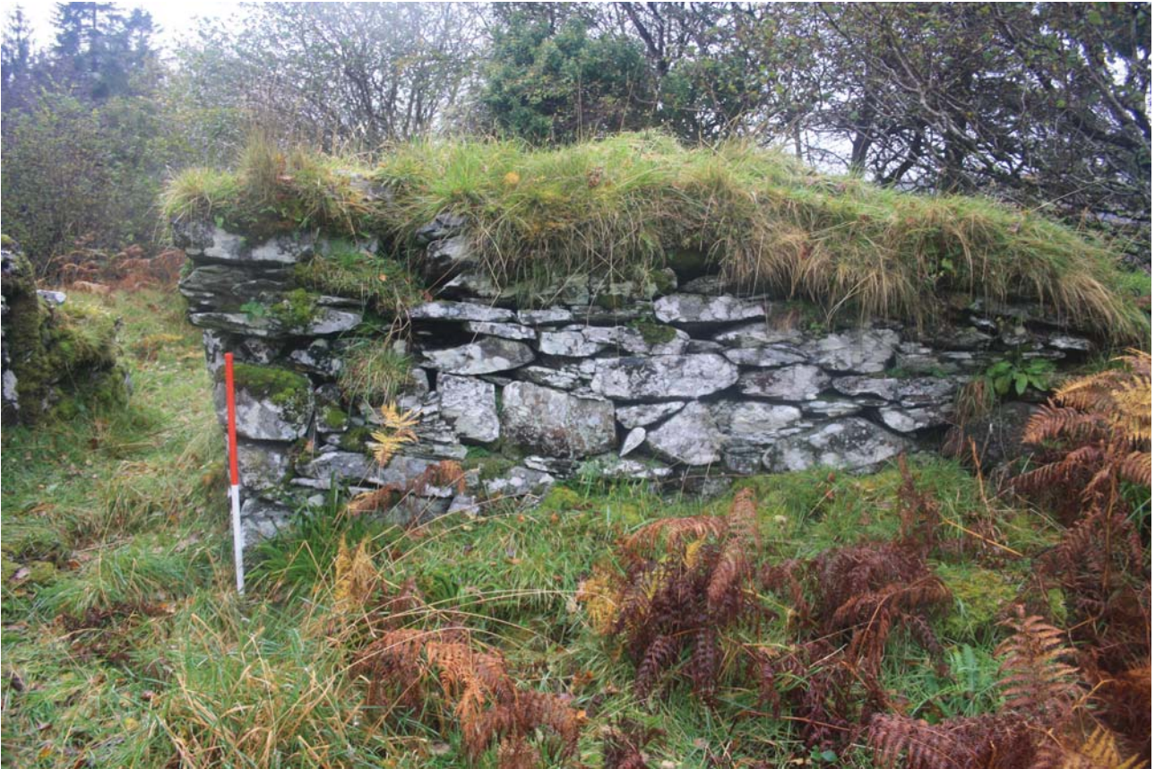
Plate 5: Internal wall face at point 3, from N
