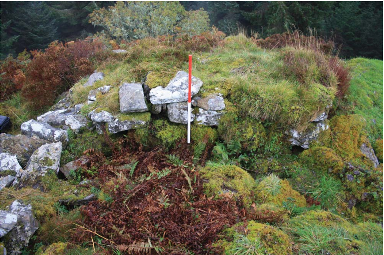
Plate 34: View of the ruinous N entrance to dun 1, at point 5, facing E
