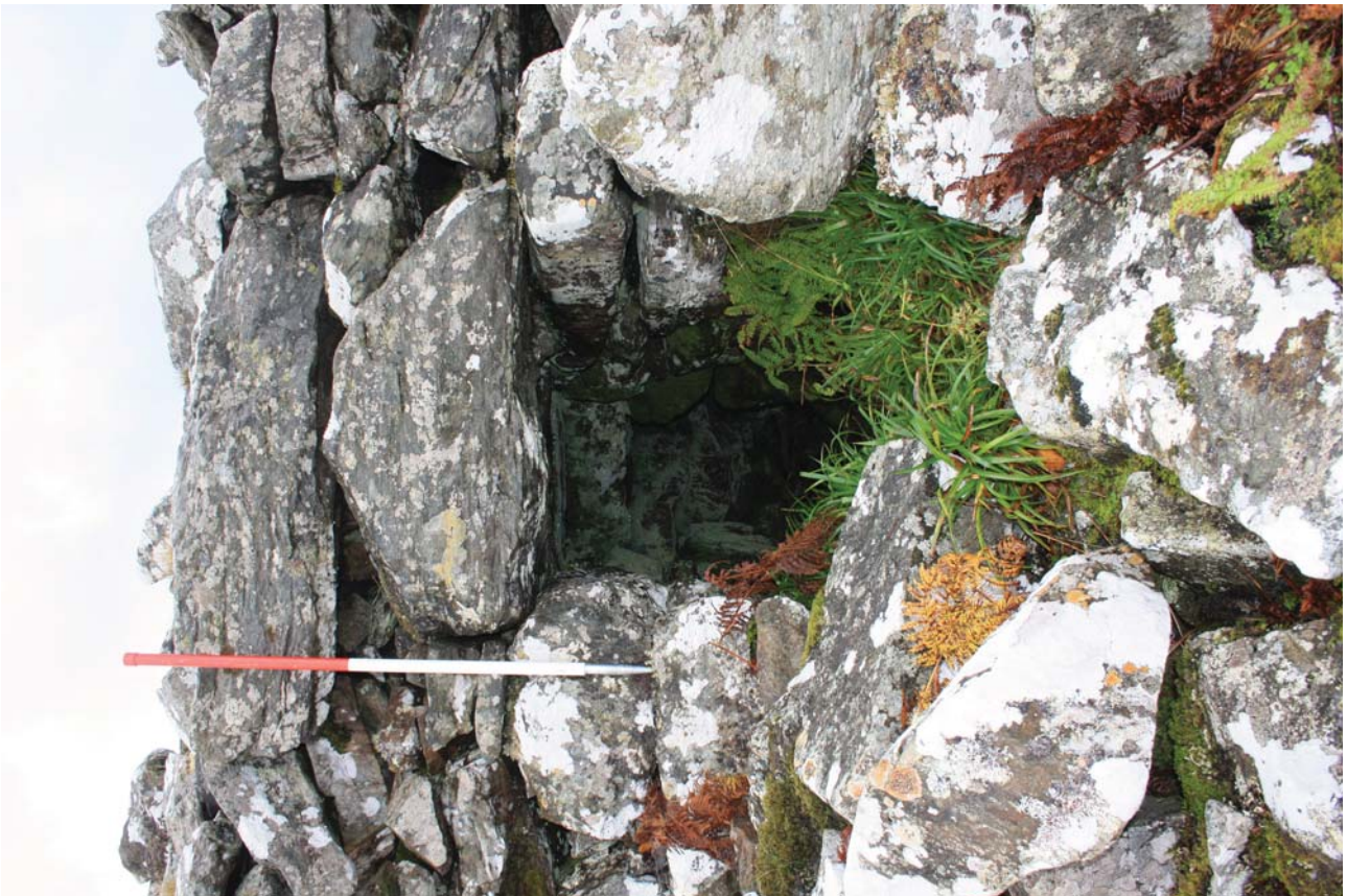
Plate 30: View into the W entrance to dun 1
