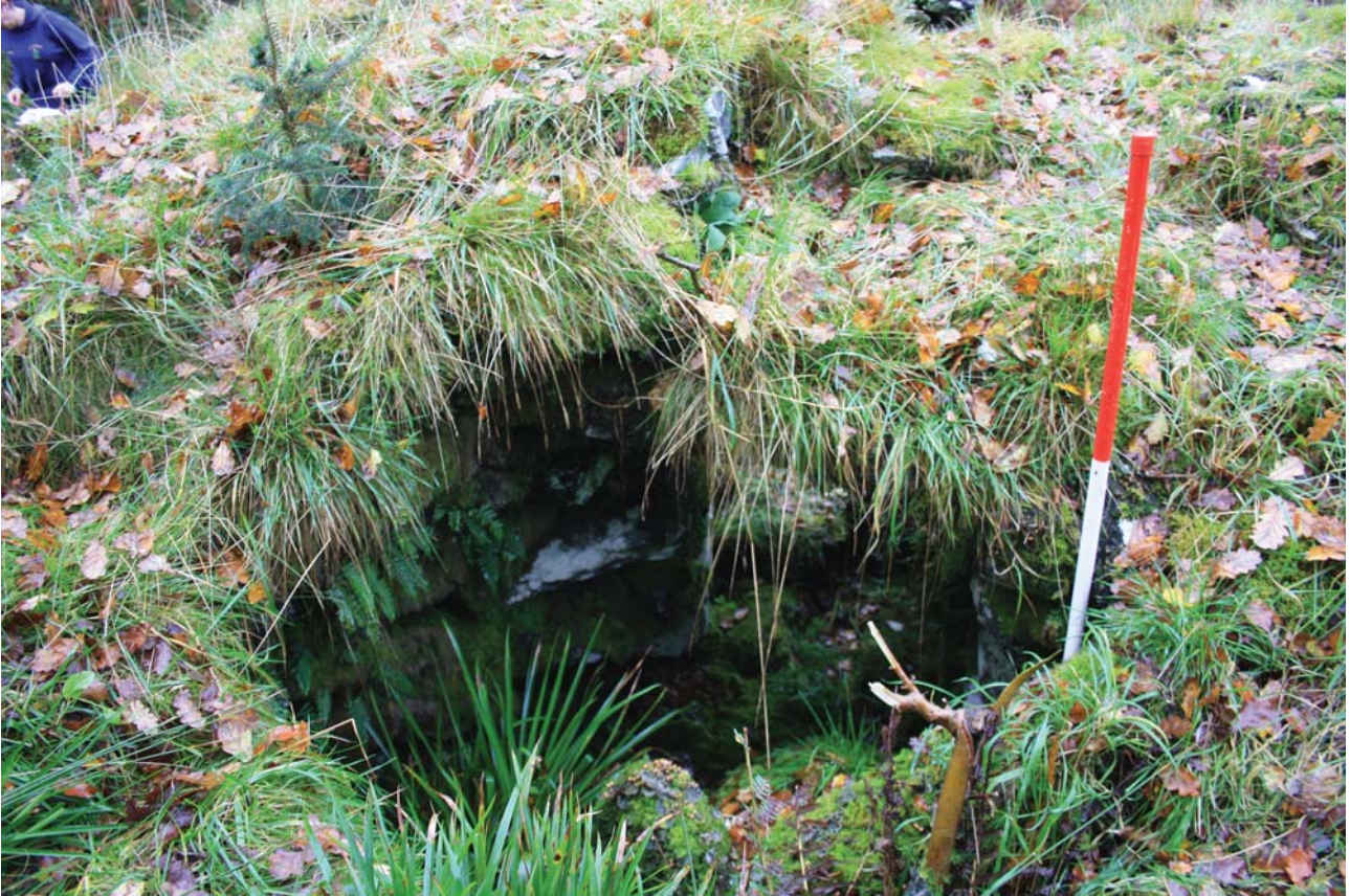
Plate 11: View into the collapsed guard cell from above, facing W
