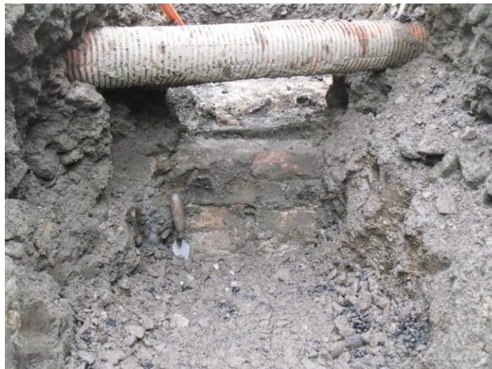
Plate 10 - Culvert [013] under the road
