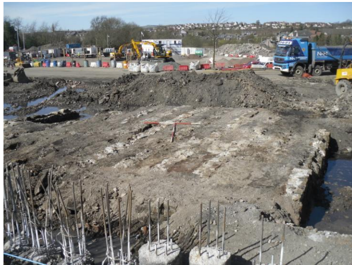
Plate 7 - Sandstone strip Foundations [034] - [042]
