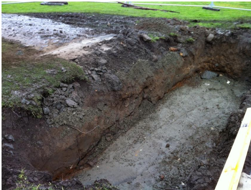
Plate1: Northern foundation trench of Peel Bridge
