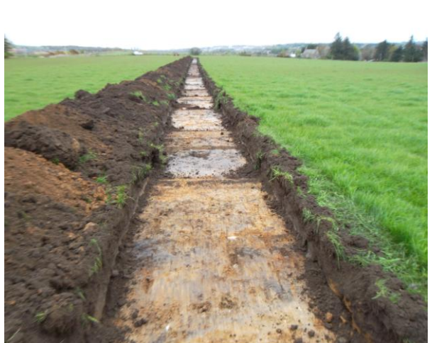
Plate 4: Trench 49 from NW
