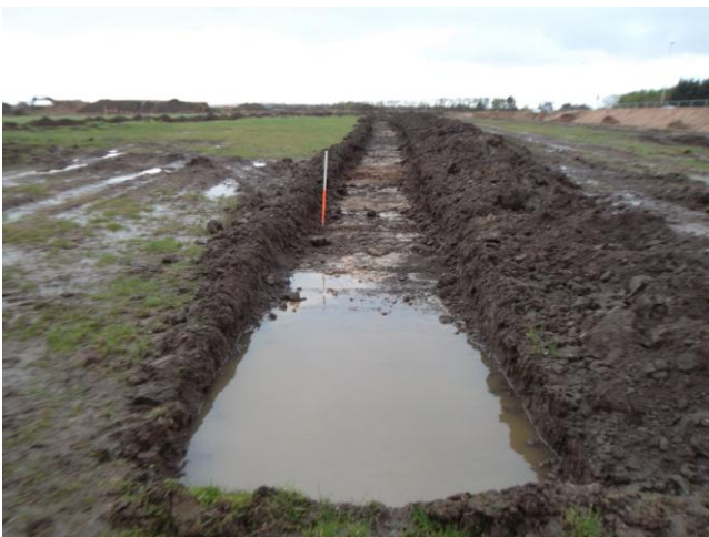
Plate 3: Trench 38 from N
