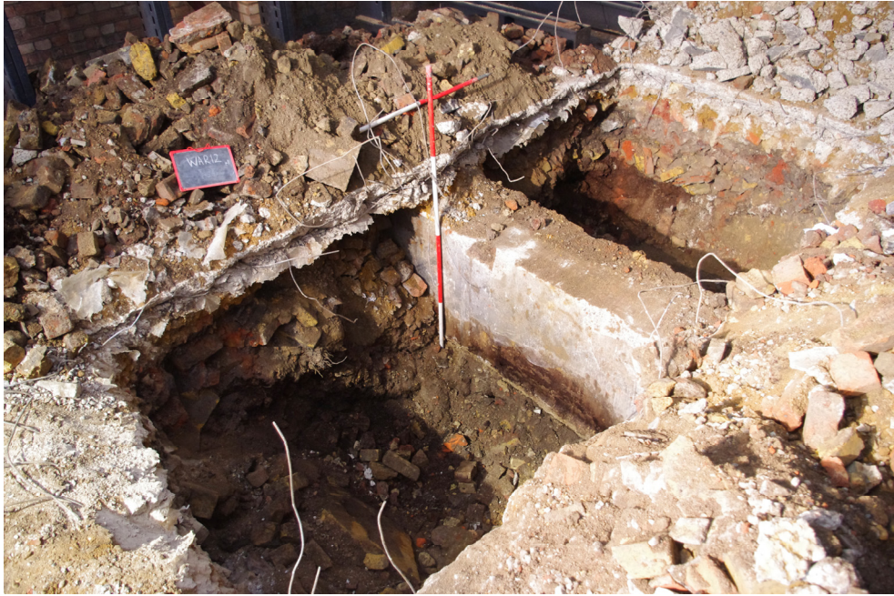
Plate 2 – Modern Concrete Footing
