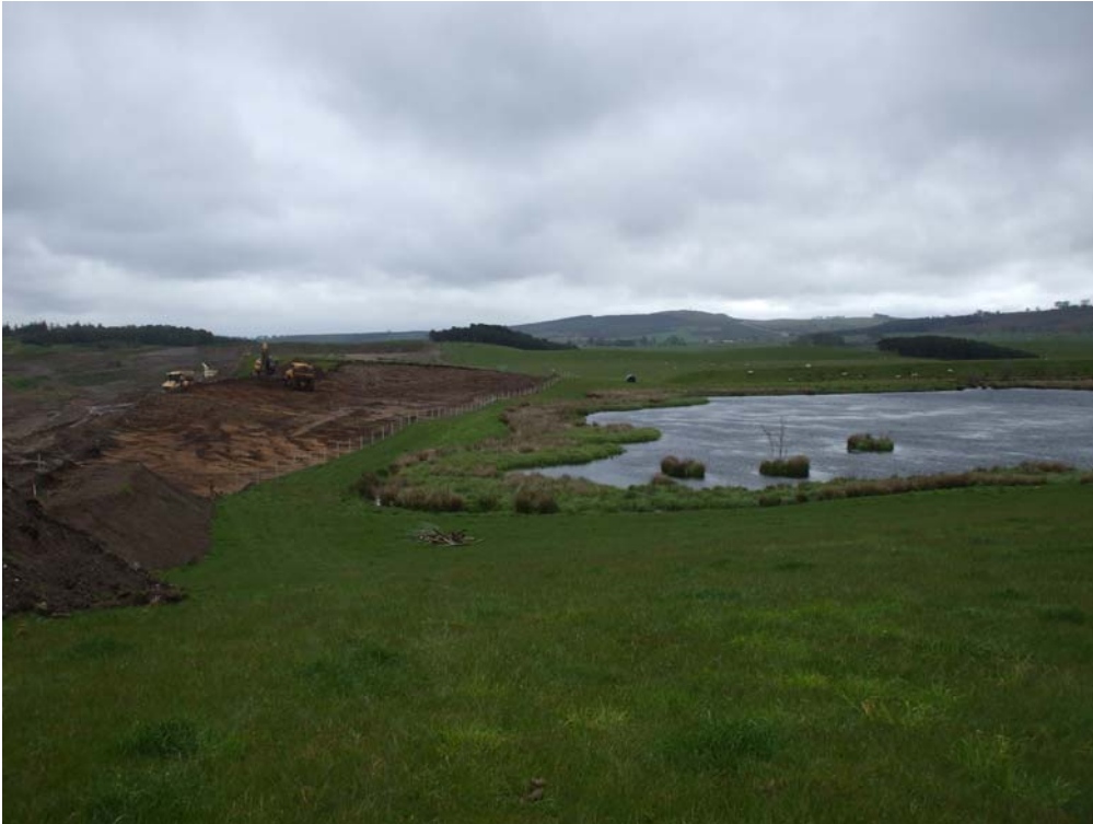
Plate 1 – General shot of stripping showing the natural pond
