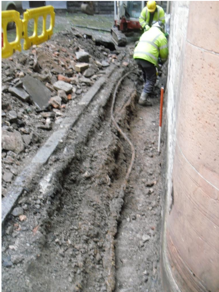
Plate 1 Trench under Excavation
