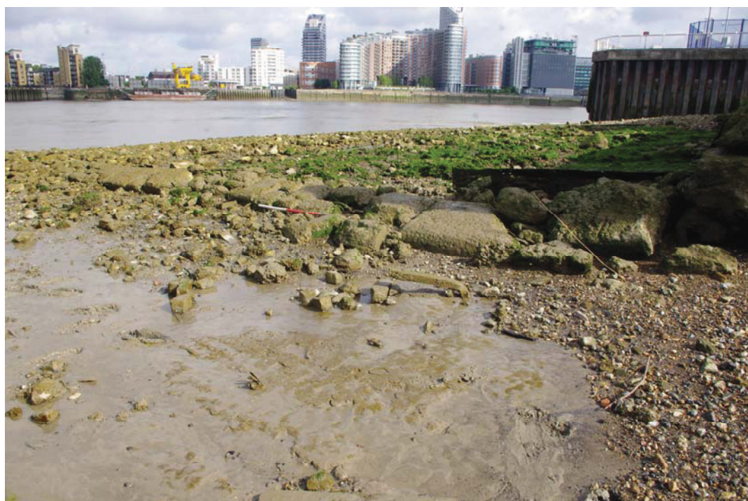
Plate 3 – Concrete wall [3] facing north-west
