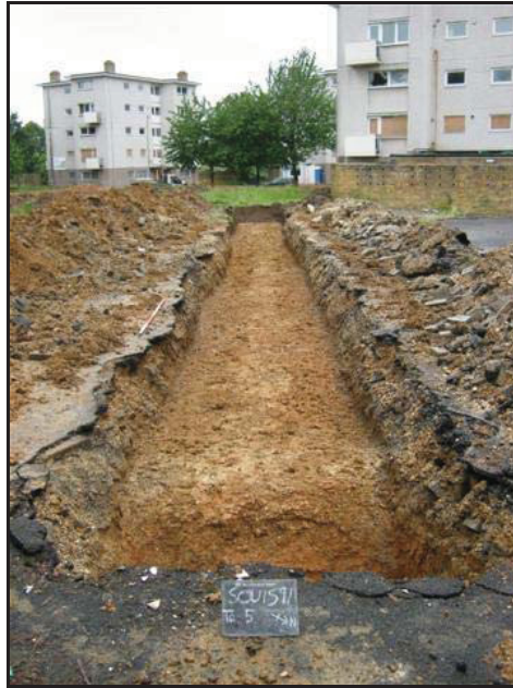
Plate E. Trench 5 Looking Southwest
