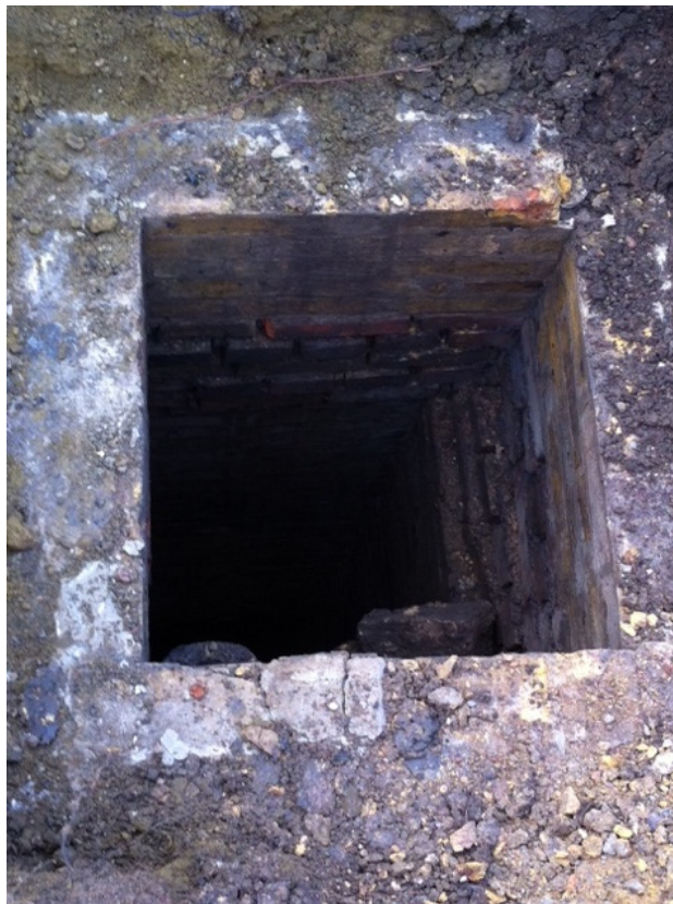
Plate 2. Inspection chamber [207], looking north
