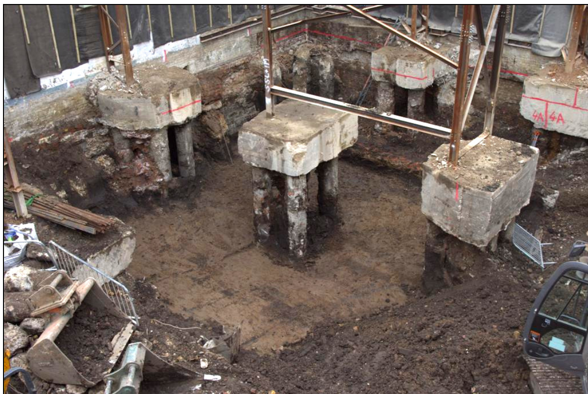
Plate 1. Site Overview looking Southwest: Brickearth with Pile Intrusions
