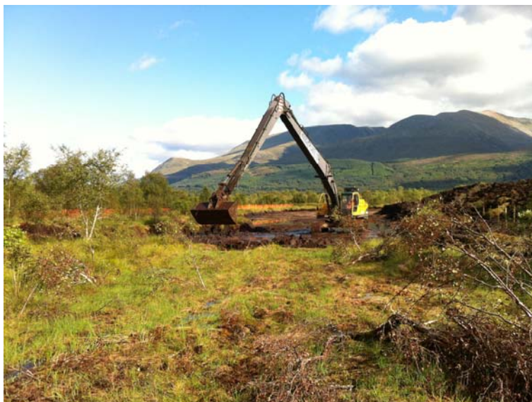
Plate 2 - Working shot of long-reach excavator on haul road
